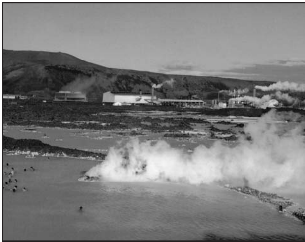
Figure 5: Blue Lagoon and Svartsengi geothermal power station
